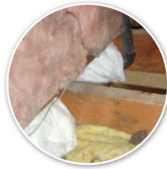
Figure 6. Air seal floor joist cavities under kneewalls by filling cavities with fiberglass batts that are rolled and stuffed in plastic bags (as shown here) or use rigid foam, Oriented Strand Board (OSB), or other air barrier board cut to fit and sealed at the edges with caulk.
